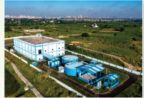
Automated Waste Collection Utility Building and Bio-Methanation Plant for waste to electricity production
